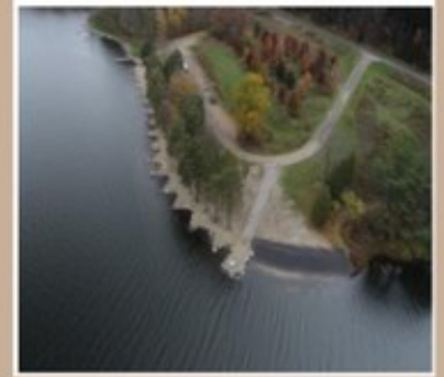
Post-Construction – Turtle Cove
