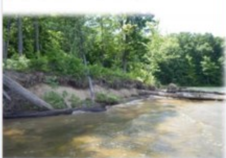
Pre-Construction – Troxel Point
