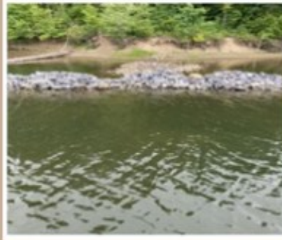
Post – Construction – Deer Inlet
