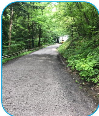
Top Section: DSA placed and rolled Bottom Section: DSA tailgated
