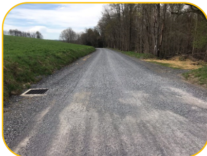
Drainage work complete and base prepared
