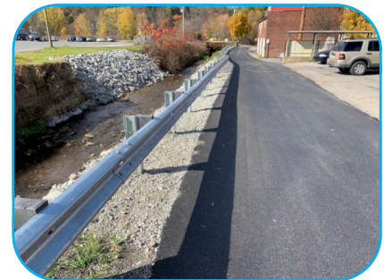
Streambank stabilized and road built back up and paved
