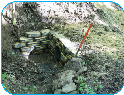
Concrete bag headwall
