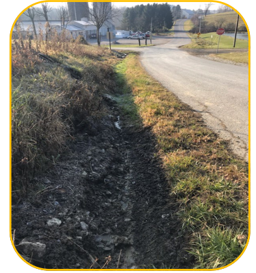
Ditch Eroding
