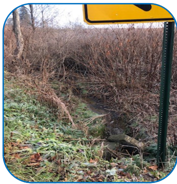
Stream crossing/ culvert replacement
