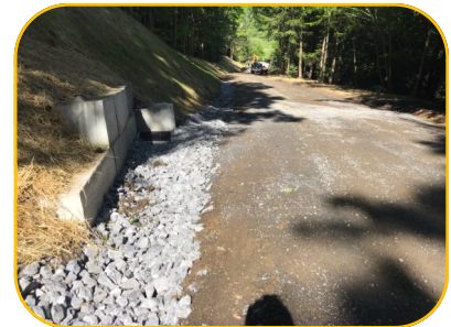
Banks laid back and cross pipes added
