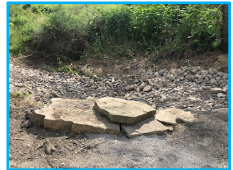
After—Headwall with R4
