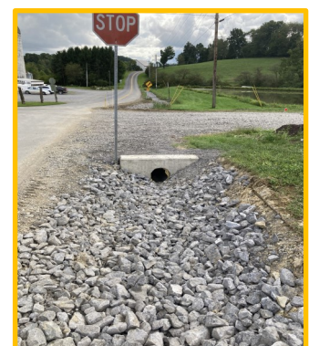
After—concrete headwall, parabola shape swale
