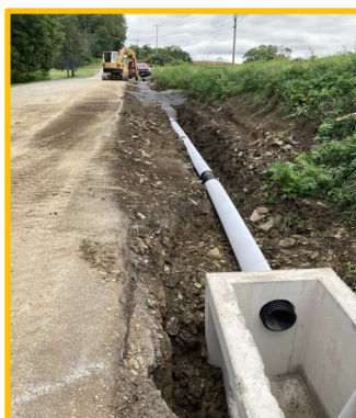
During construction—underdrain with geofabric
