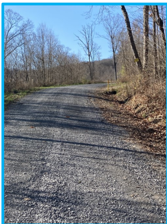
After—driveway pipe, headwalls & endwalls, 2A to build up road base
