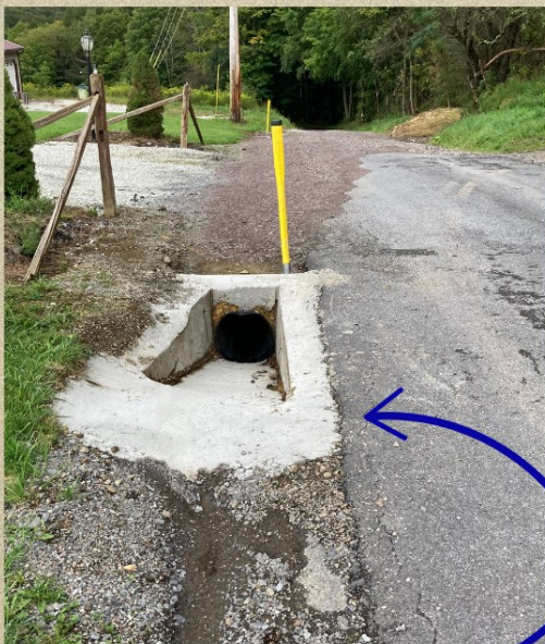
Concrete headwall of cross pipe
